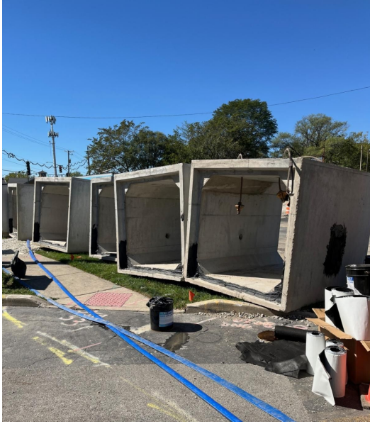
Box culvert installation
