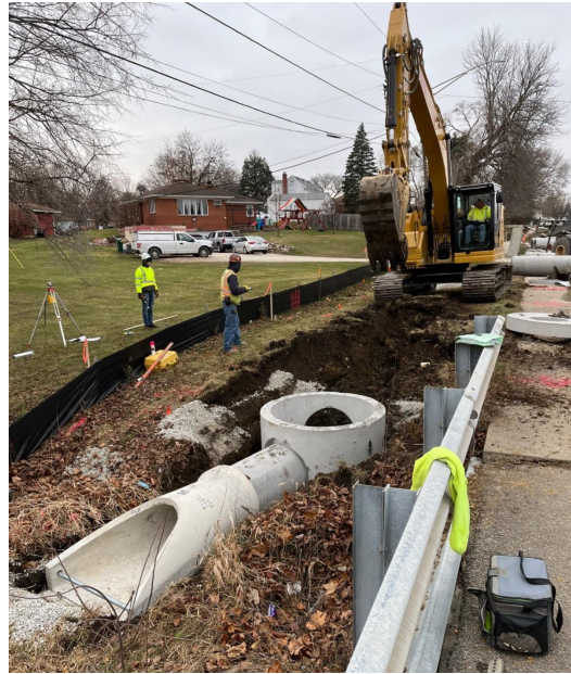
Storm sewer installation
