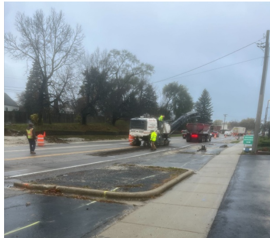
Pothole Patching with Hot Mix Asphalt
