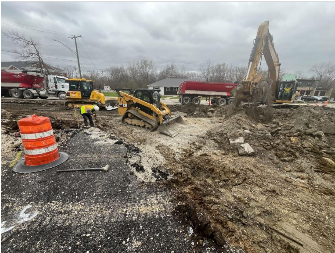
Pavement removal
